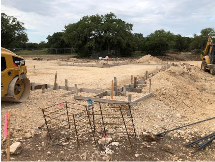
Prep for Concrete Slab and Grade Beams
