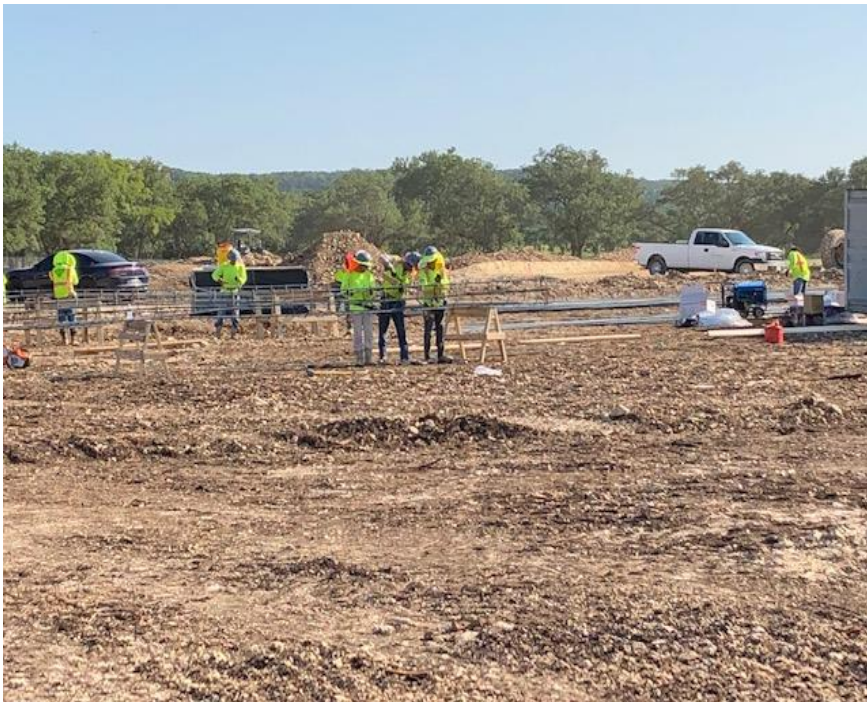
Drilled Pier Reinforcing Prep
