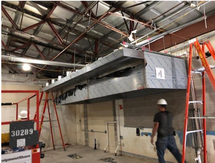
Kitchen Exhaust Hood Installation
