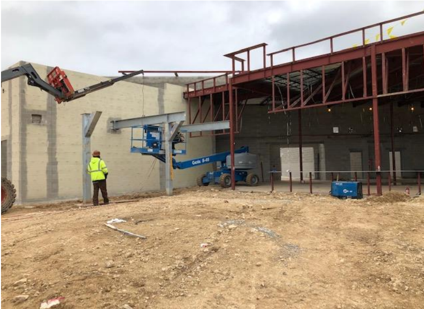
Canopy Framing at Main Entry
