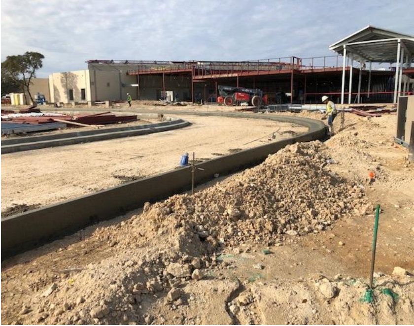
Main Entrance Drive Curb Placement
