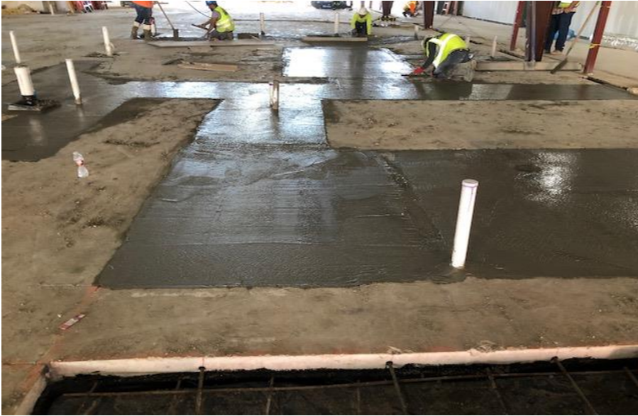
Underfloor Work and Concrete Replacement at Annex
