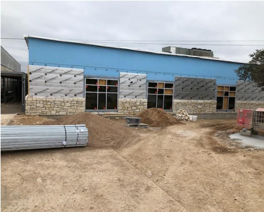
Exterior Masonry and Window Installation Classroom at Addition
