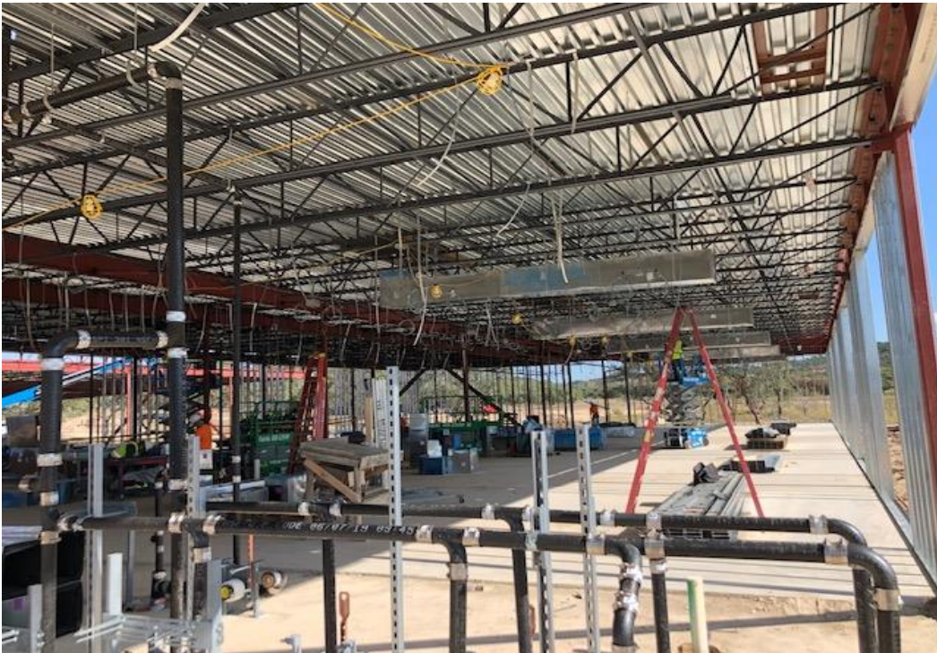
Interior Wall Framing and HVAC at Classroom Area A
