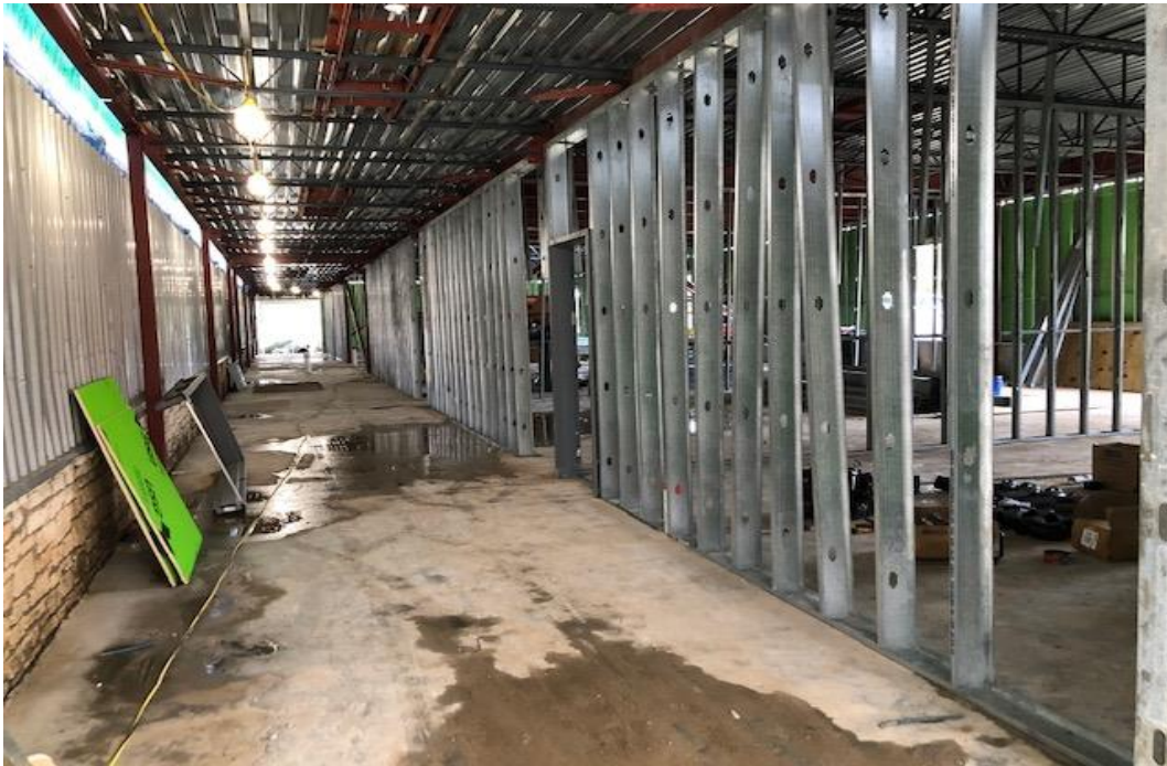
Classroom Addition Interior Wall Framing
