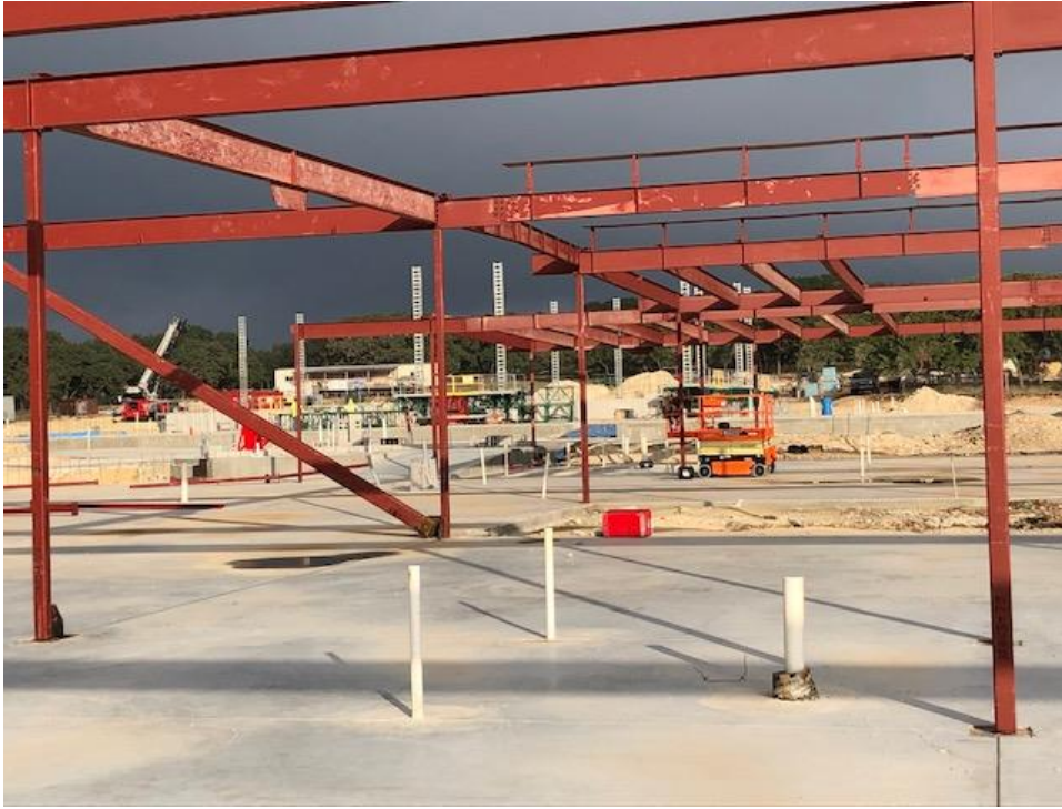
Structural Steel Erection at Classroom Area A
