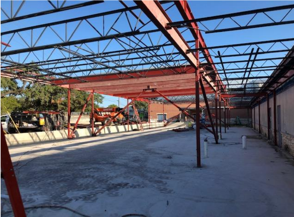
Classroom Addition Structural Framing
