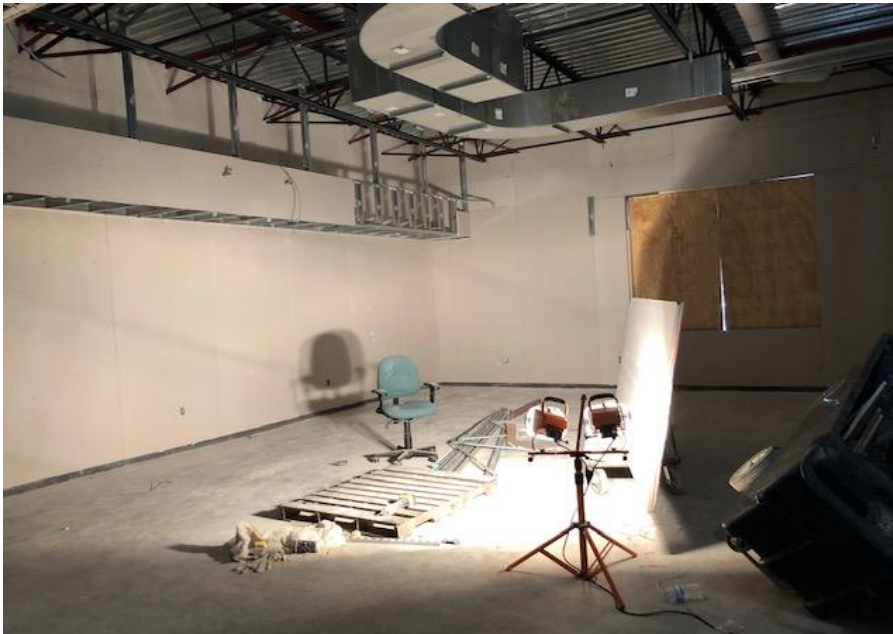
Typical Classroom at Addition
