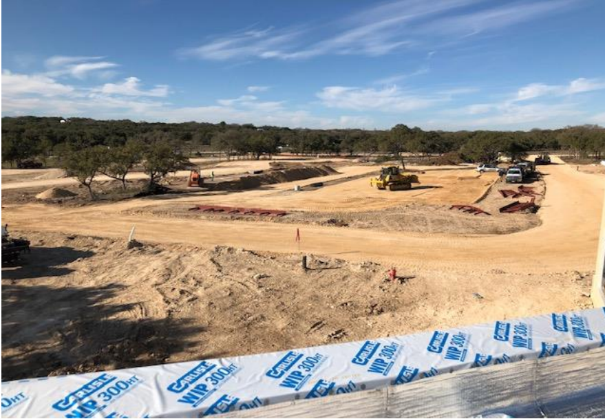
Rooftop View Front Parking Lot
